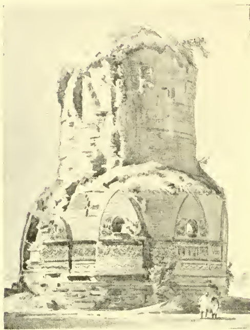
THE DHAMÊKH TOWER
